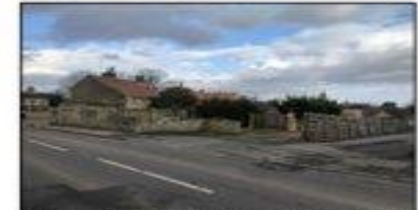
Corner Cottage, existing flat roofed extension, boundary fence and boundary wall viewed from the southwest
